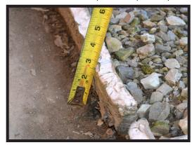
This insulation was placed on the exterior of the 4' frost footing. Each spring, approximately 2-3" of insulation has to be removed as the frost has pushed it up.
